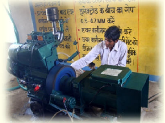
Local Operator of Biogas Engine
