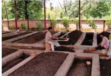
Overground brick lined compost pit
